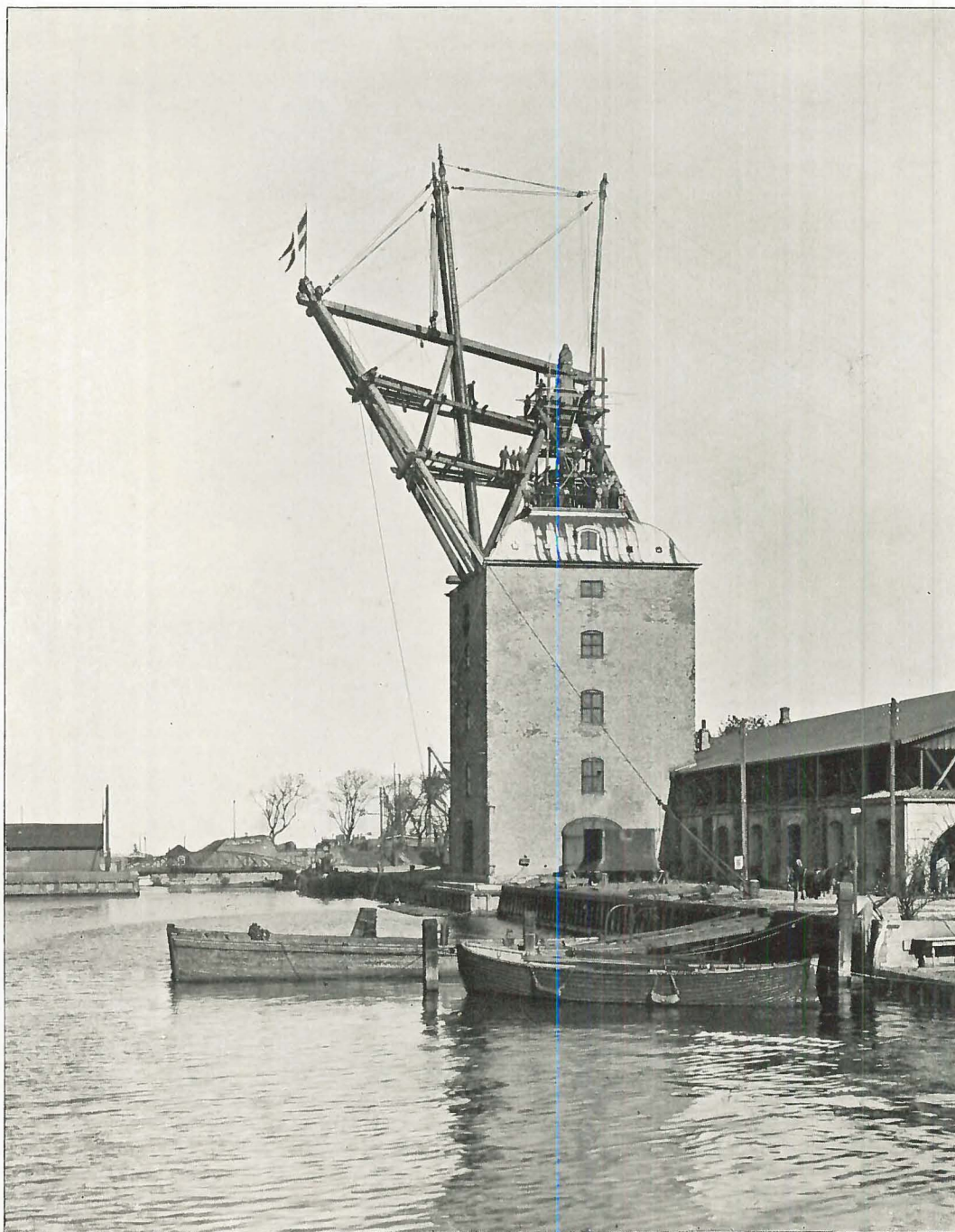
Nyholms Krans Hovedreparation, 1922.
