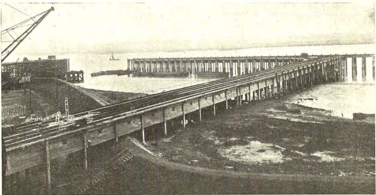
Discharging bridge on the Thames, Depth of water 11 mtr.
