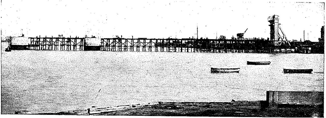
Landing - jetty at Harwich-Ferry »Harwich-Zeibrugge«.
