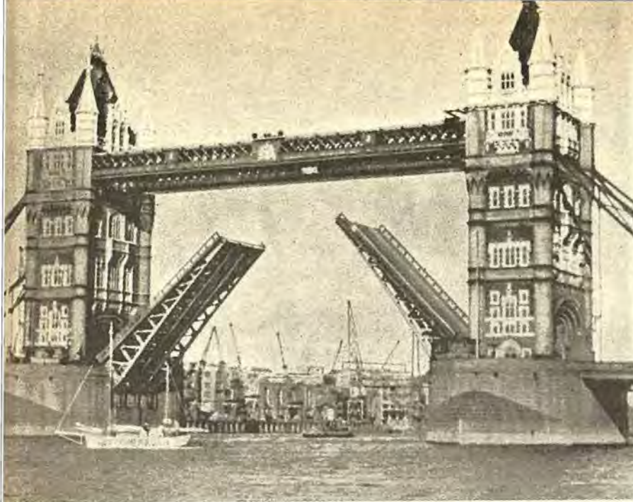
„Idle Hour“ passerer Tower Bridge.
