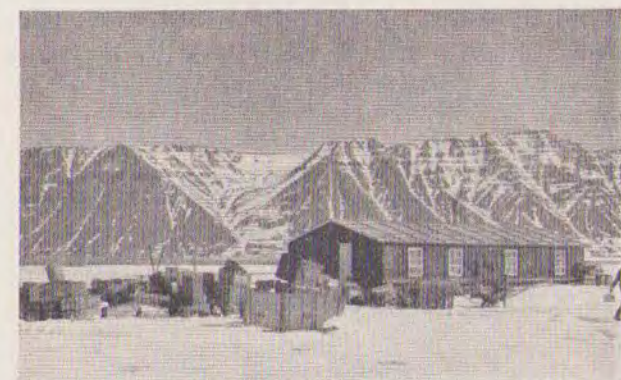
En Decca-station under etablering.
